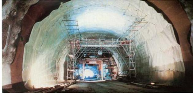
**Figure 1.** Trenchless two-shell tunnel with geomembrane sealing during construction
