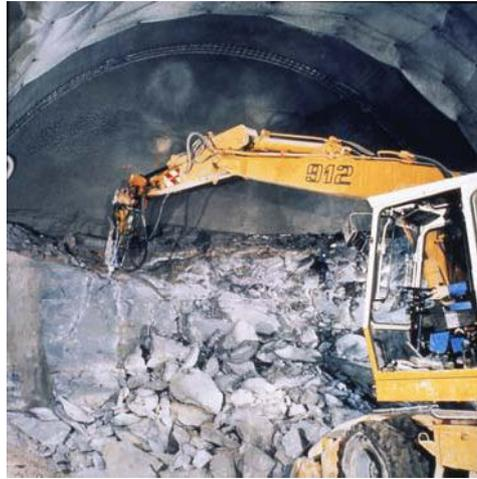
Fig. 9: Excavation work of the frozen bulkhead
