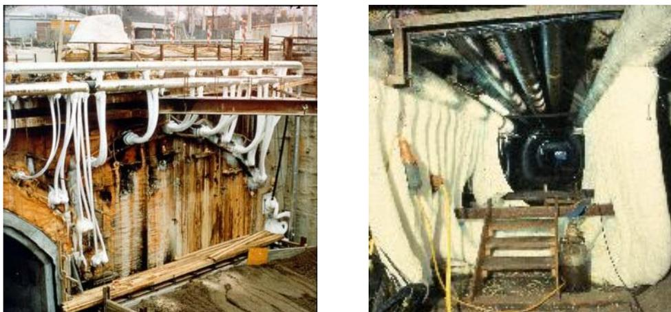
Fig. 8: Installation of freezing hoses
