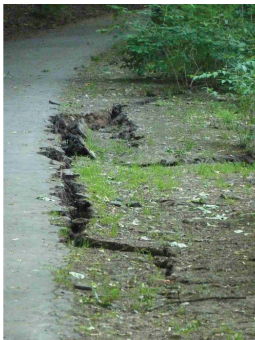
Fig. 1. Longitudinal crack on the surface of the clay core – Jirkov dam. Fig. 2. Tensile crack at the upper part of slope.
