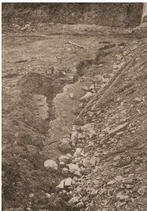
Fig. 1. Longitudinal crack on the surface of the clay core – Jirkov dam. Fig. 2. Tensile crack at the upper part of slope.
